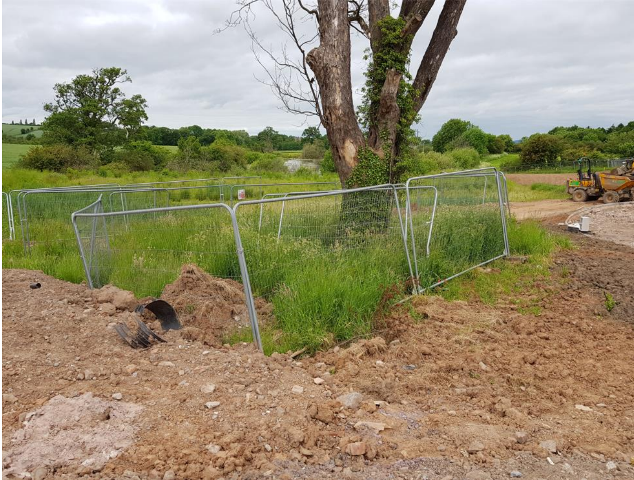
10 th of June 2021 T15 Sycamore. According to the tree protection plan. The fencing should have been set out at 12.2 metres from the trunk.
